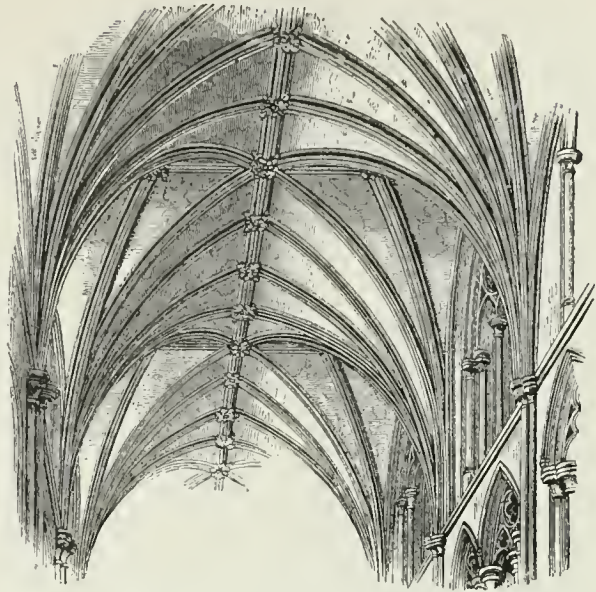
RIB, FIG. 2: VAULTING OF 1260 WITH MANY RIBS USED FOR ORNAMENT ALONE, AS THOSE AT THE RIDGE OF THE VAULT, AND ALL THE OTHERS NOT FOUND IN FIG. 1; WESTMINSTER ABBEY.
